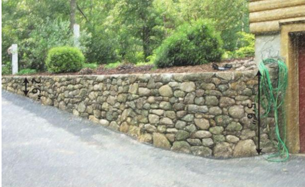
Figure 3-05. Retaining Wall Height
